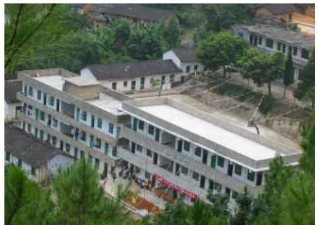
The new 3 storey Changping Central School building
